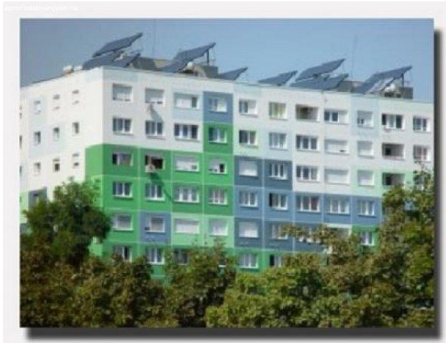
„ECO-housing estate” in Budapest
